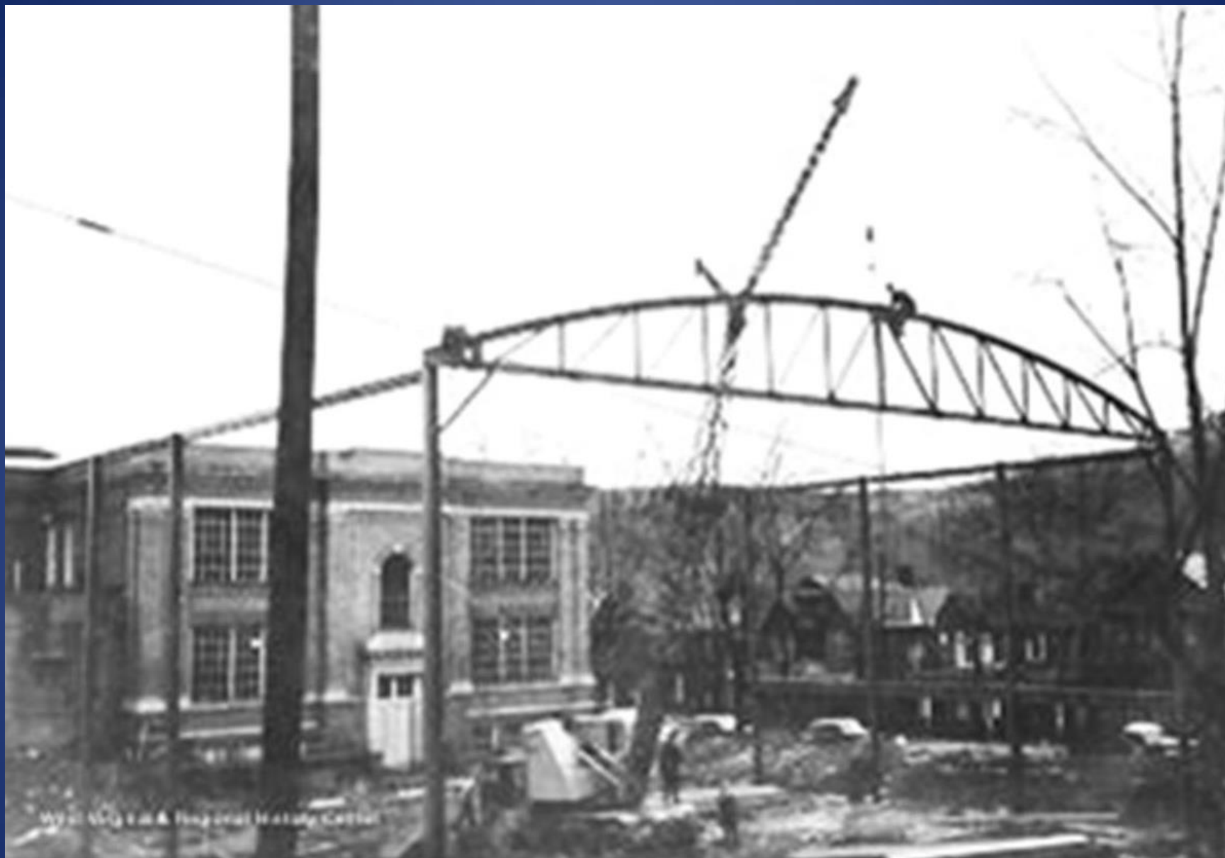
Early Construction of the Perry Memorial Gym - 1952
