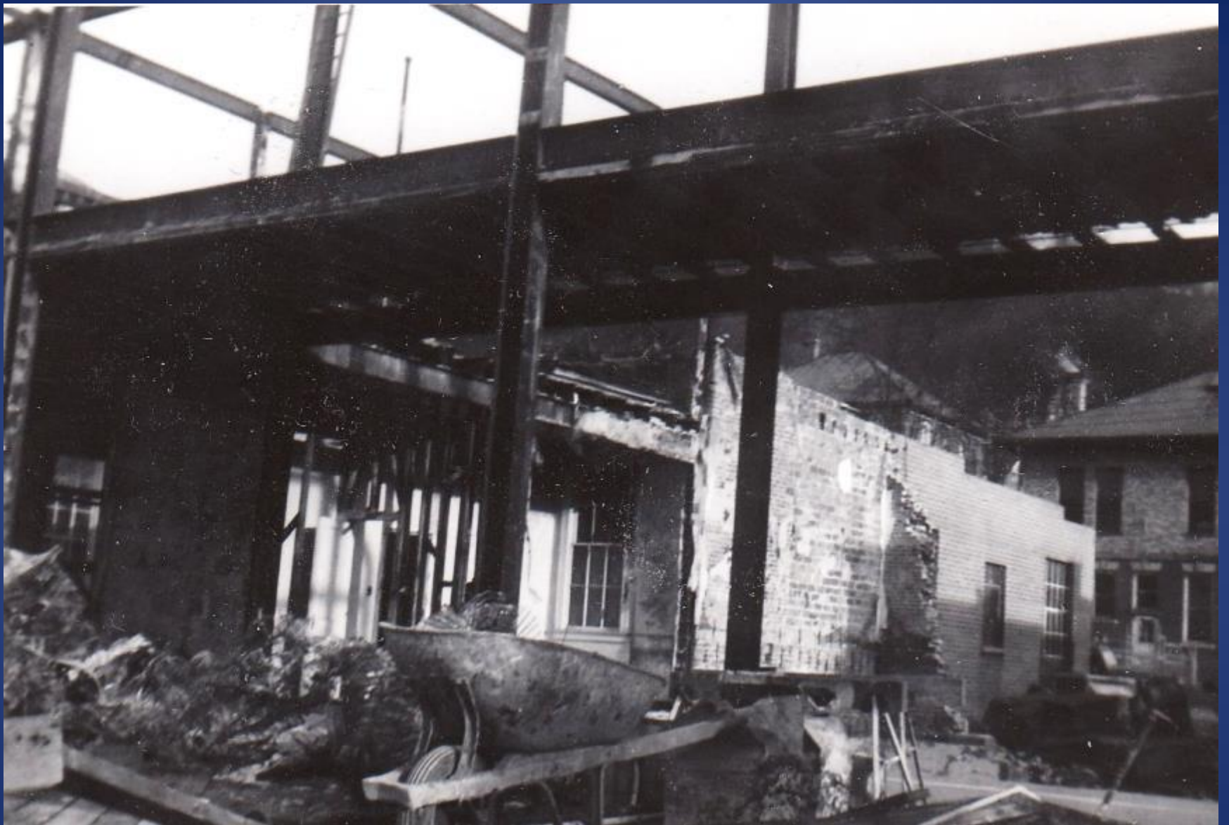
Results of Hinton High School Fire Notice Library Building on Ballengee Street
